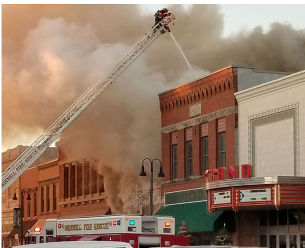
The fire at 915 Main that left the lot in a state of disrepair. Photo Credit: KCRG.
