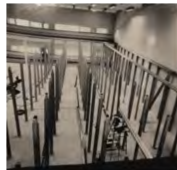
Construction photos of the "top hat" addition
